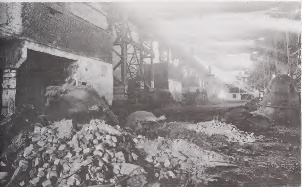
A power plant for a textile mill complex on the outskirts of Tiranë Courtesy Charles Sudetic Elbasan Steel Combine Courtesy Fred Conrad
